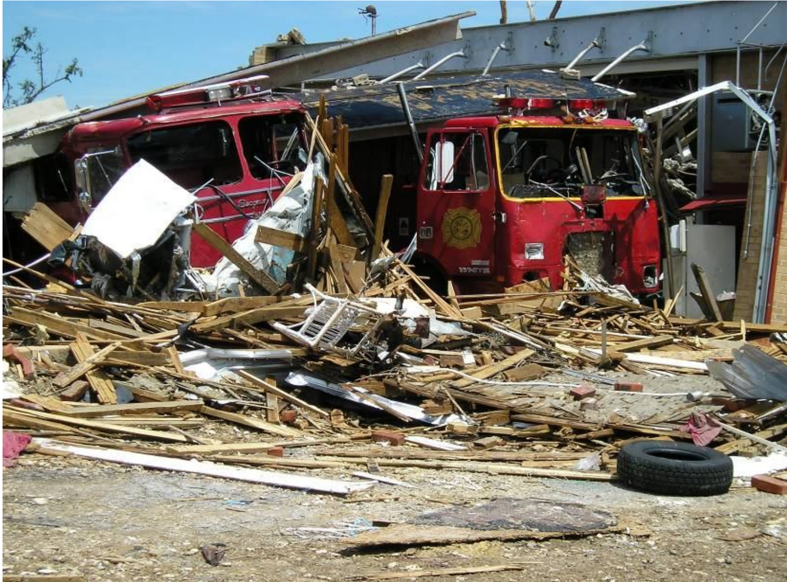
Greensburg, KS, Tornado, May 2007 – photo courtesy USAR TF-3
