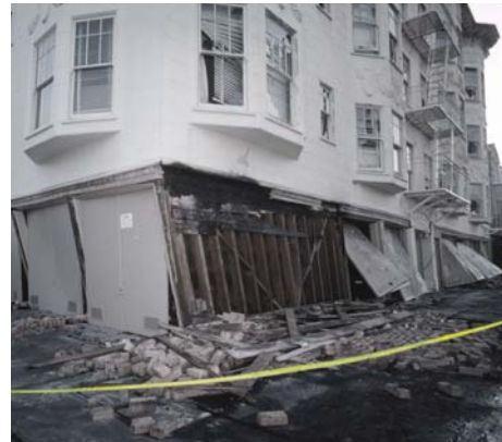
“Soft story” buildings, typically with parking on the ground floor, like the one pictured here, are common throughout the Bay Area and are particularly at risk when exposed to strong shaking (USGS photo).
