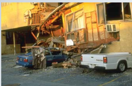
The first story of this apartment building collapsed, crushing cars below (FEMA photo).
